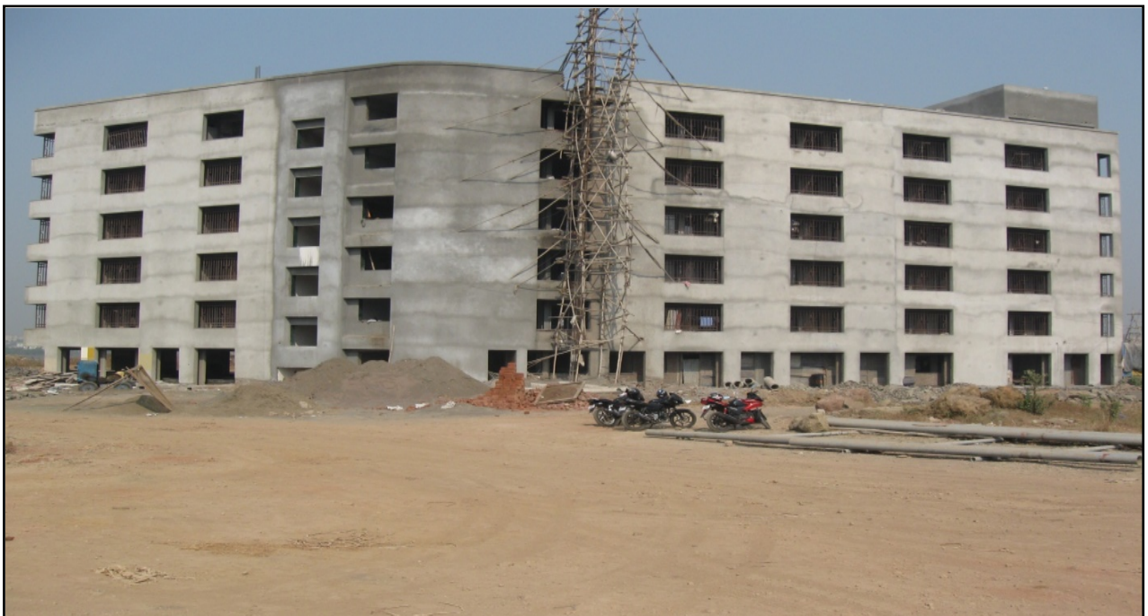
Hostel Building Rear View
