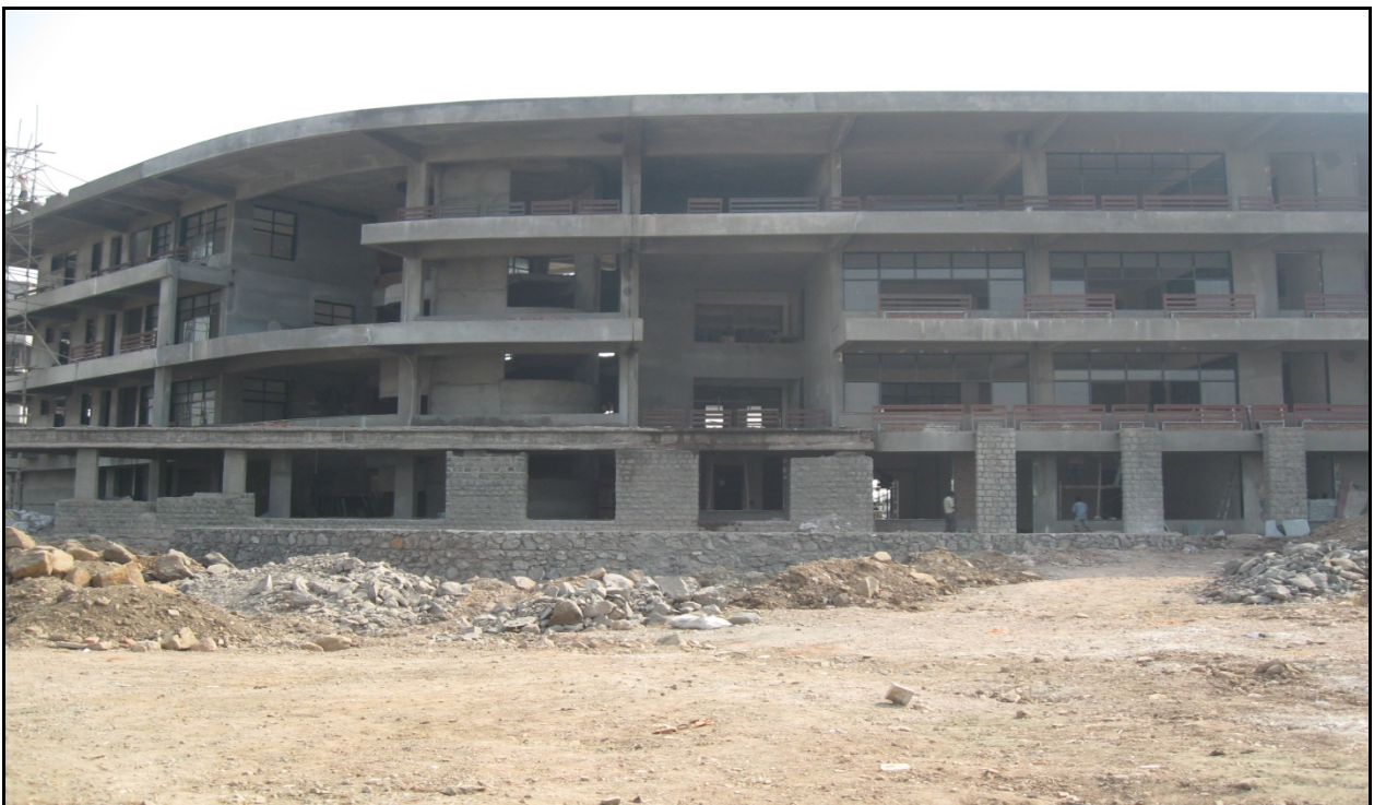
Permanent Building Rear View
